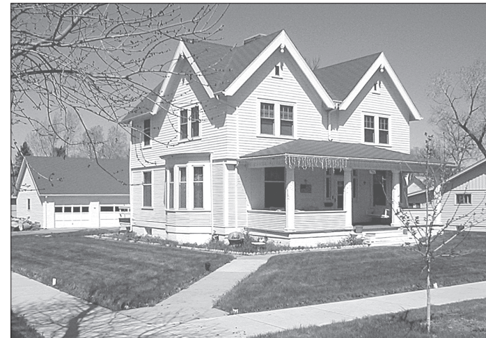
Kidwell House, looking northwest.
