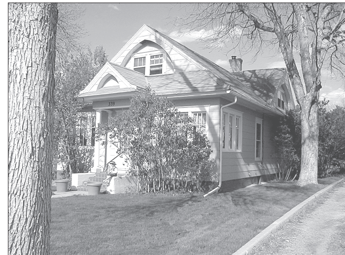
Rice House, looking northeast.
