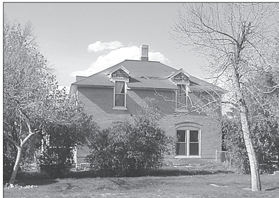
Cook House, looking north.
