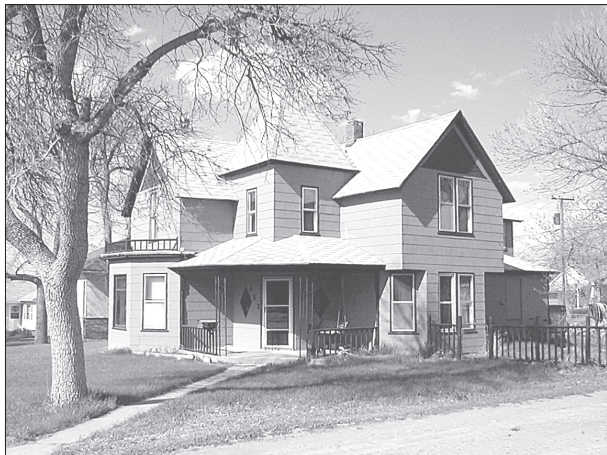
McWhinnie House, looking northeast.
