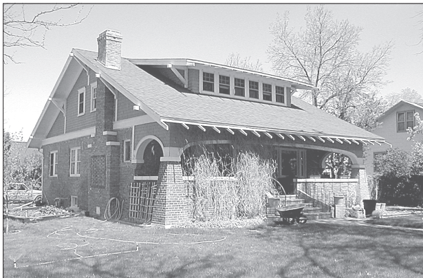
Garst House, looking northeast.
